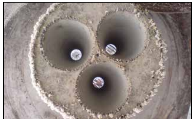
Inside the unit is clean and fully operational.
