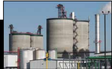
Nebraska Ethanol Plant
